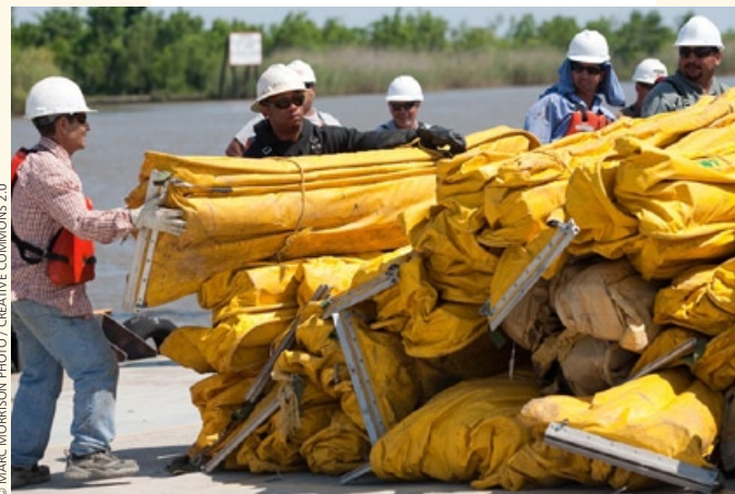
U.S. Environmental Service workers deploy containment booms to aid in oil cleanup in the gulf.
